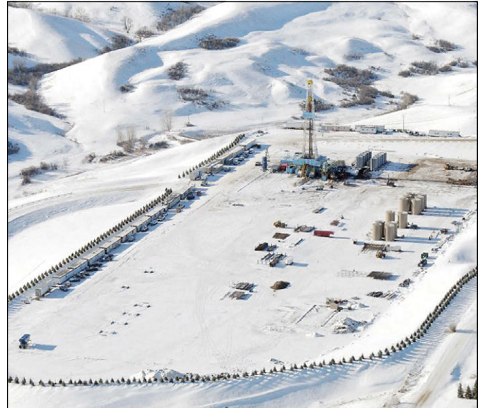
This is an aerial view of the Continental Resources 20-acre drill pad where an all electric drilling program is being used for the 14 wells on the outskirts of Williston near the Missouri River.
